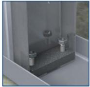
Fasten anchors to floor with specified washers.
